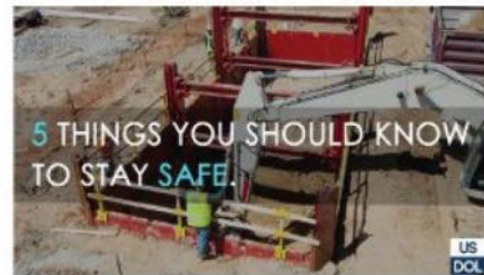
Trench Safety PSA ▶▶
